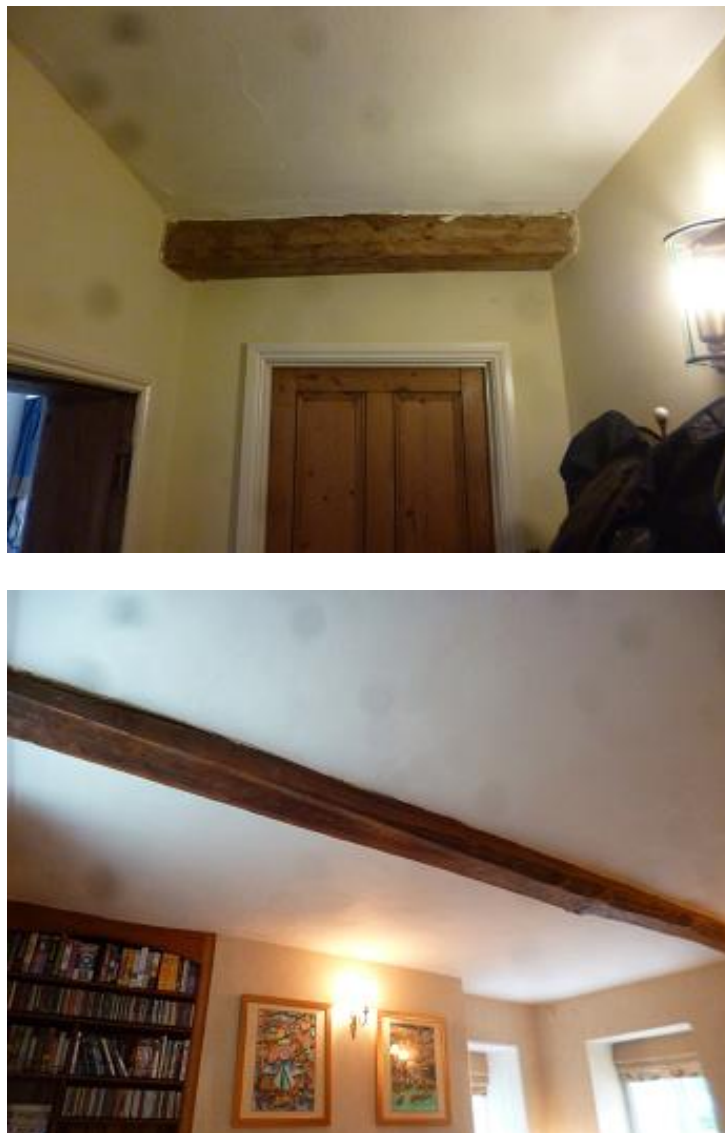
Figure 7: View of timbers at Holme Farm
