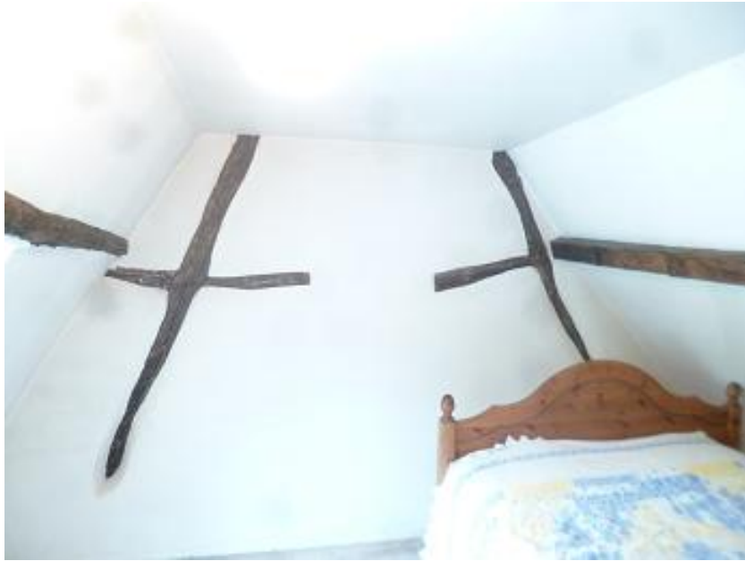
Figure 9: View of timbers at 20 Mill Lane
