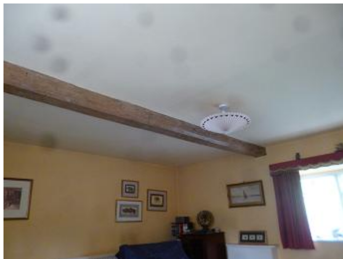
Figure 5: View of the timbers at Honeypot Cottage
