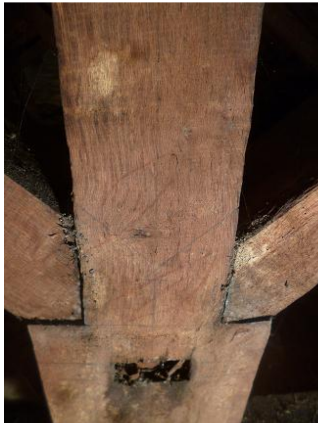
Figure 10: View of the roof trusses at the Grange (top) and detail of the marking-out lines and other markings in red on a king-post (bottom)
