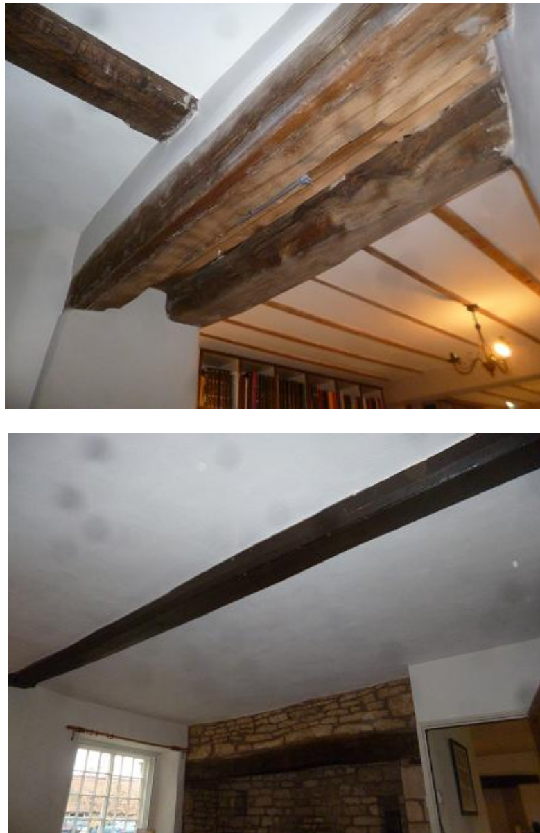
Figure 6: View of timbers at Fir Tree Farm
